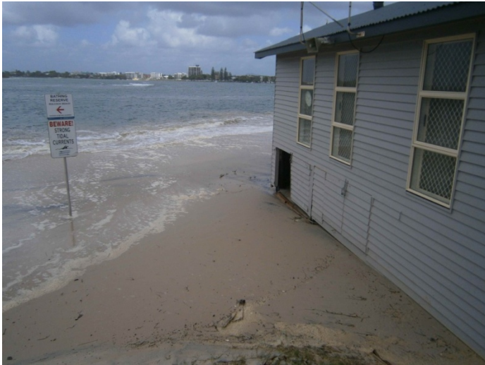
January 2011 cyclone, high tides & clubhouse threatened
